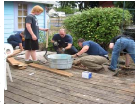
Repairing the ramp
